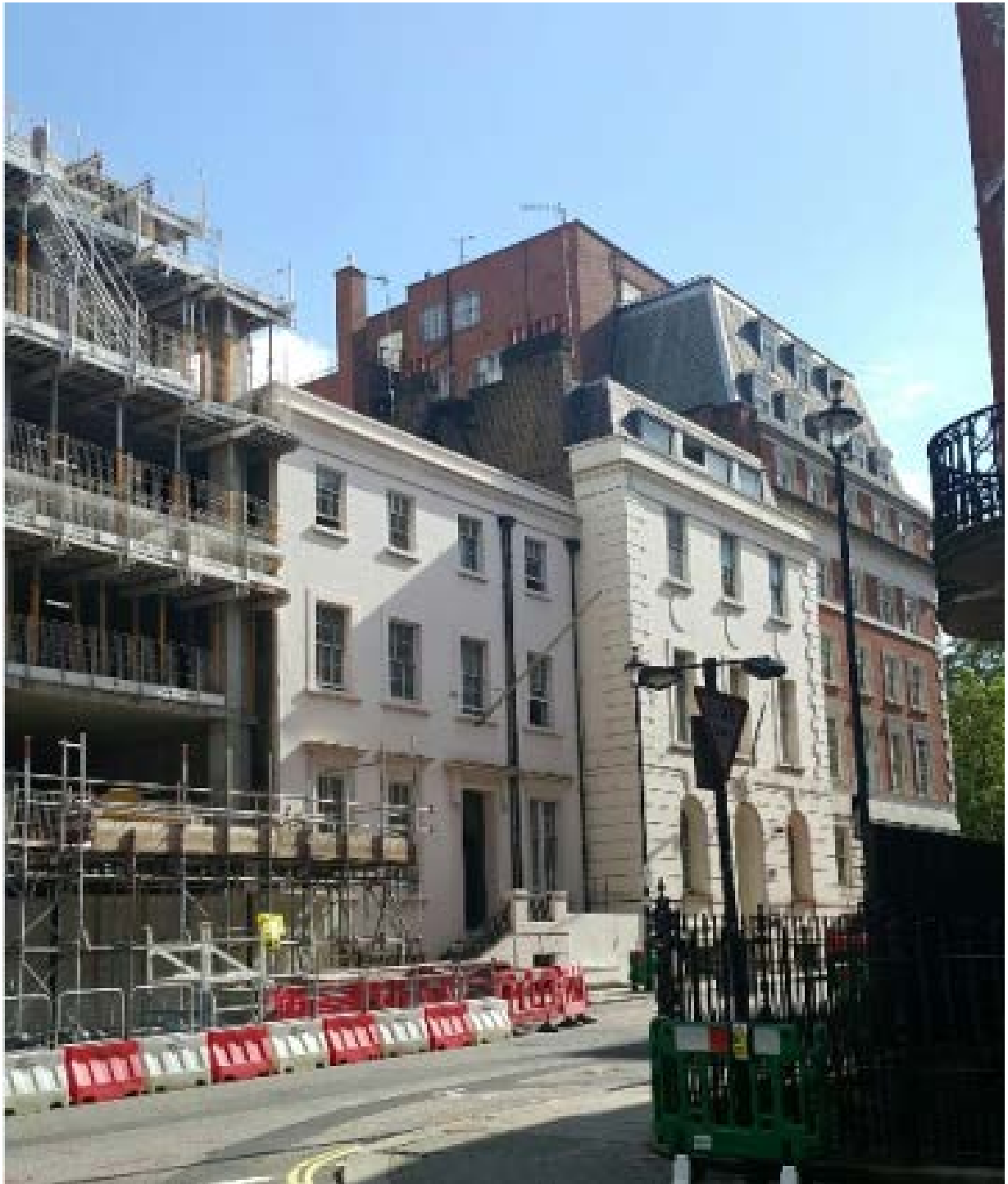
Site 1: 75-77 Brook Street
